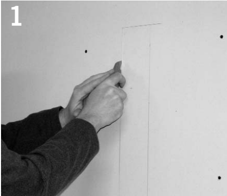
1 Cut hole in drywall per dimensions shown.
