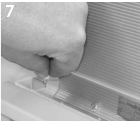
7 Remove screws from glass to lamp fixture. (where applicable)
