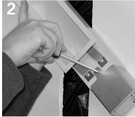
2 Remove electrical box cover from fixture.
