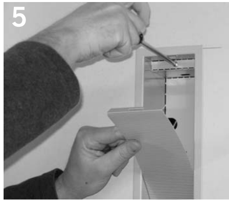
5 Pop reflector out and tighten screw to secure fixture into wall. (N/A for ZTO)
