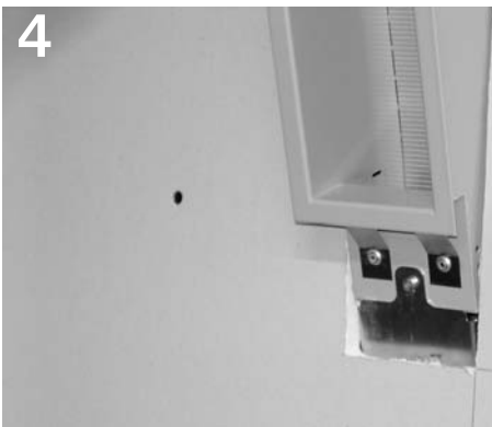
4 Replace electrical cover and install in wall.
