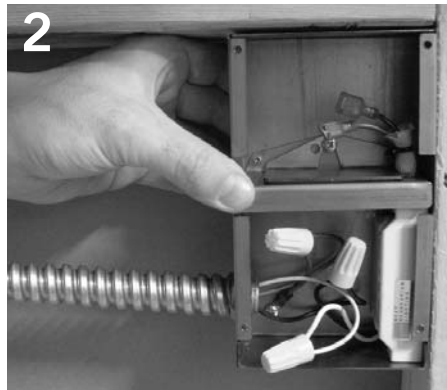
2 Connect conduit and make electrical connection to primary wires from LED driver.
