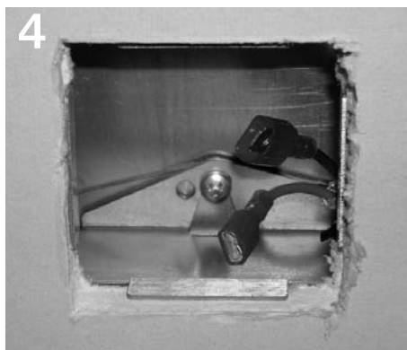
4 Install wall board. Cut hole in drywall around opening in Zas wall box (approx. 2.25" square).
