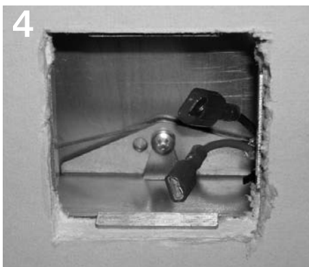
4 Install wall board. Cut hole in drywall around opening in Zas wall box (approx. 2.25" square).
