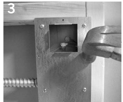
3 Reattach wall box cover by replacing (4) screws and attach box to stud wall.
