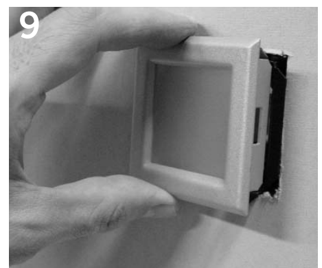
9 Snap LED housing lens cover into fixture housing. Fixture should be flush to wall when complete.
