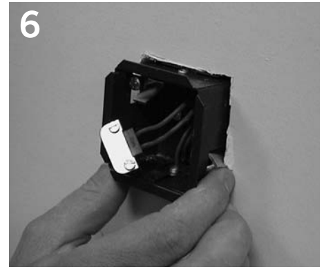
6 Snap housing into backbox.
