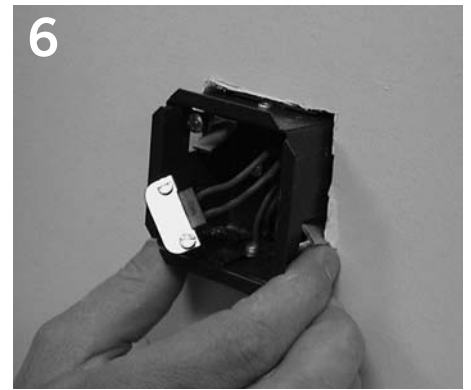
6 Snap housing into backbox.
