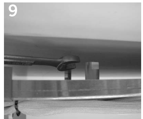
9 Prior to tightening mounting screws, base may be leveled to ceiling by adjusting mounting feet with 13mm wrench (not included).
