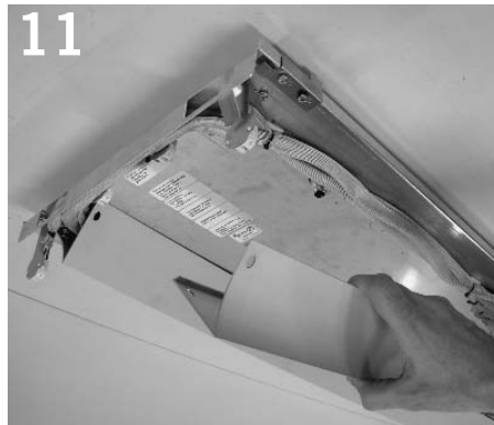
11 Re-install reflectors and tighten screws. NOTE: Curved side of reflector should face outboard, as shown.
