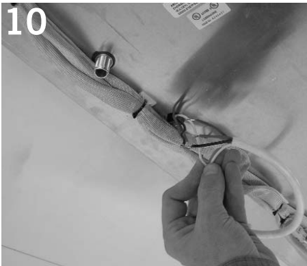
10 Make electrical connection. Push wires and connectors back into junction box.
