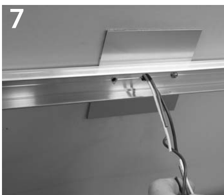
7 Make electrical connection.
