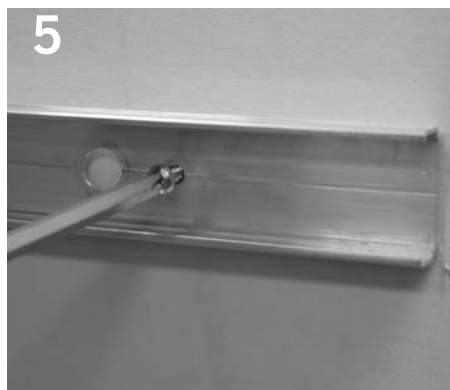
5 Screw channel back to wall.
