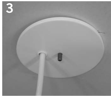
3 Make electrical connection in j-box and slide canopy over 1/4-20 stud.
