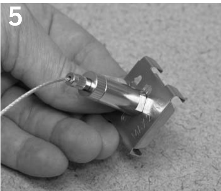
5 Slide cables into cable grippers.
