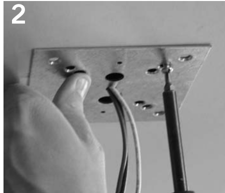
2 Secure mounting plate with two counter-sunk screws.
