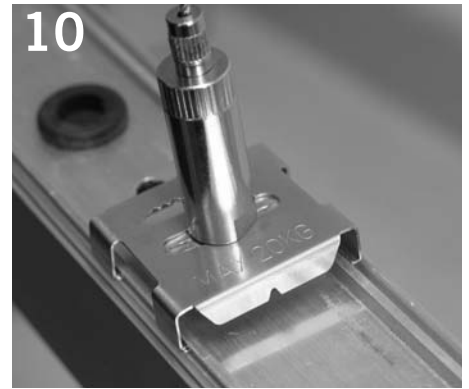
10 Slide cables into cable grippers.
