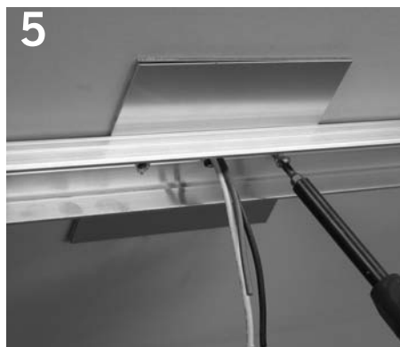
5 Secure channel back to mounting plate with 2 screws.
