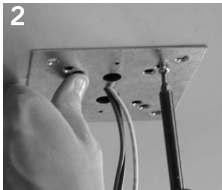
2 Secure mounting plate with two counter-sunk screws.
