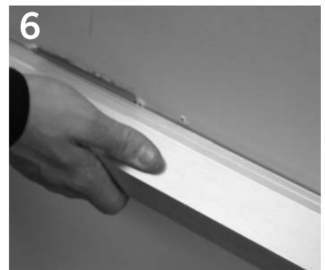
6 Snap fixture onto channel back.
