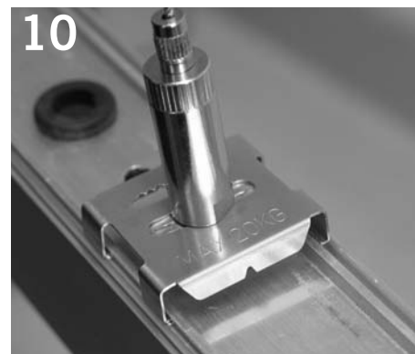
Slide cables into cable grippers.
