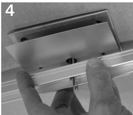
4 Insert building supply wires through center hole in trim plate and through center hole in back channel. Trim plate should be between back channel and junction box plate, as shown.
