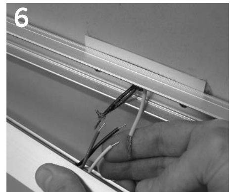
6 Make electrical connection.
