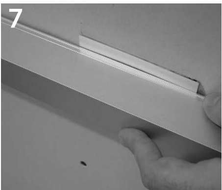
7 Snap fixture onto back channel.
