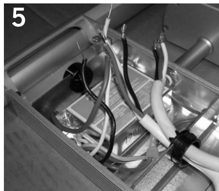
5 If continuing circuit to additional modules, thread cord in from opposite direction and make electrical connection in metal electrical enclosure.
