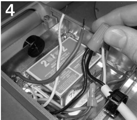
4 Make electrical connection inside metal electrical enclosure.
