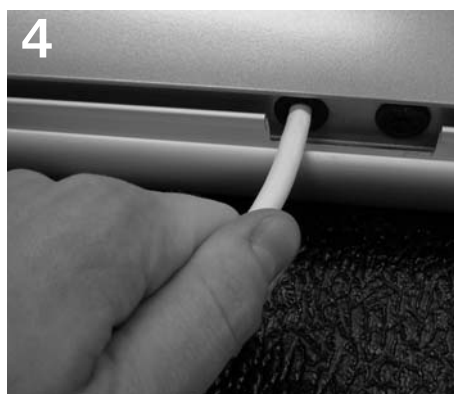
4 Remove tube cover and feed incoming SJT from Tube through one hole in side of fixture. If continuing circuit, feed outgoing cord through second hole.
