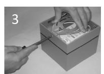
Detach mounting plate from fixture by removing screws in fixture.
