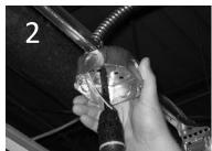
If using a T-grid ceiling, attach the octagonal /Energie J-box to the Caddy/B-Line bar as shown. If installing in a hard ceiling mount the j-box to structure. Run conduit to J-box with proper feed wiring for that location.
