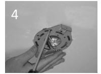
Attach mounting bracket to junction box
