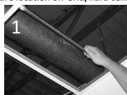
If using a T-grid ceiling, attach the Caddy/B-line crossbar to the T-grid ceiling as shown. Make sure to tie the crossbar off to the ceiling structure per code.
