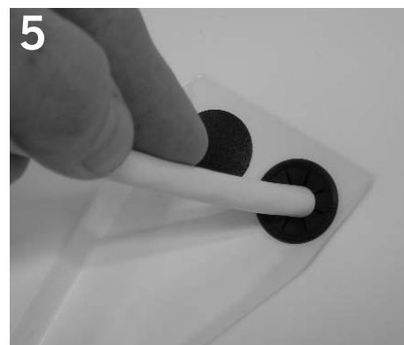
5 Raise luminaire up to j-box and pull cord through the bushing as shown.
