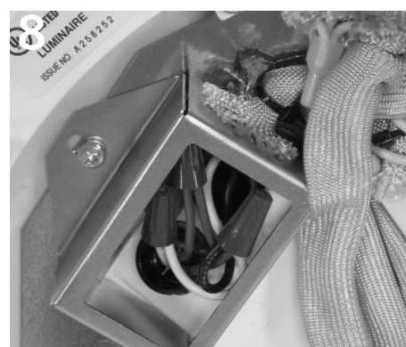
8 Push connections into splice compartment in luminaire.
