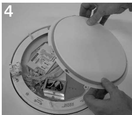
4 Remove ballast cover by loosening (3) screws and turning cover counterclockwise.
