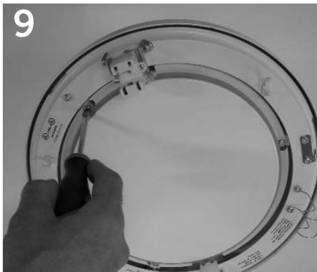
9 Replace ballast cover and tighten securing screws.
