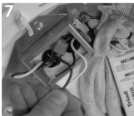
7 Trim excess cord and make electrical connection inside luminaire.
