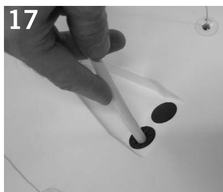
17 Insert lower end of power cord into bushing on top of luminaire.
