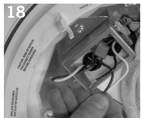
18 Trim excess cord and make electrical connection inside luminaire.
