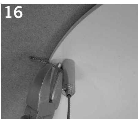
16 Trim excess cable at grippers.
