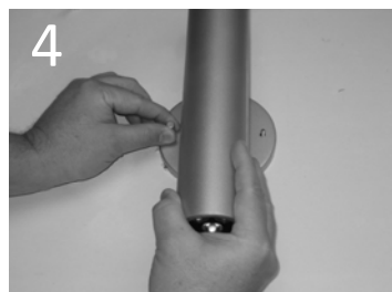
4 Align fixture mounting bracket to the fixture and secure with supplied thumb screws.
