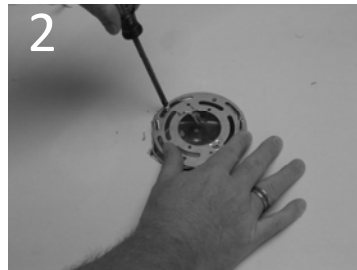
2 Run supply wires from wall through supplied mounting bracket and attach the mounting bracket to the octagonal J-box.
