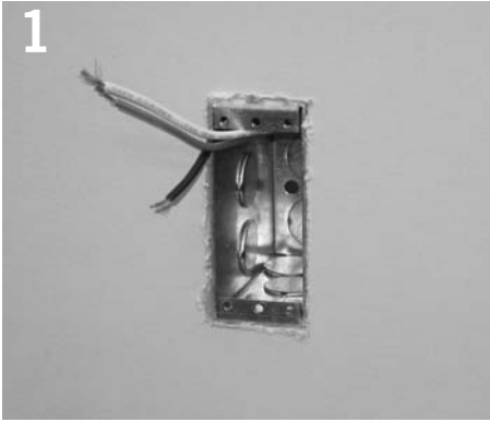
1 Install Energie junction box vertically into wall.
