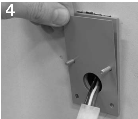
4 Slide coverplate over mounting plate.
