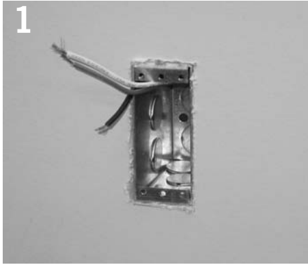
1 Install Energie junction box vertically into wall.
