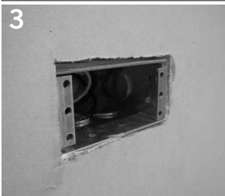
3 Install Energie junction box horizontally into wall.
