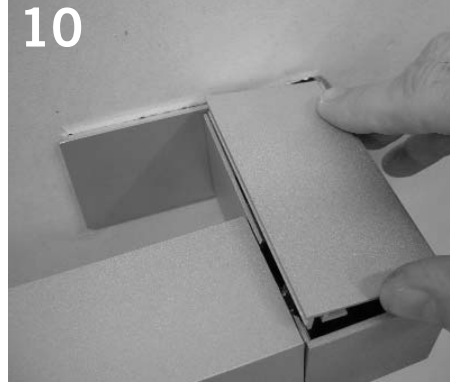
Snap end block covers into place. NOTE: Cover lip should face wall.
