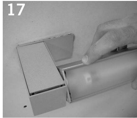
17 Rotate luminaire body to desired orientation.
