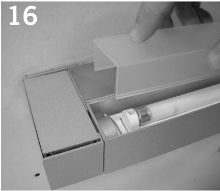
16 Remove diffuser and install lamp per relamp label. Replace diffuser.
