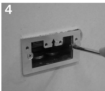
4 Install mounting plate onto junction box using (2) #8-32 FH screws (provided). NOTE: Orient mounting plate with arrow pointing up.
