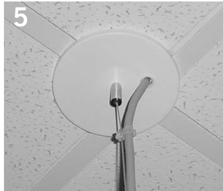
5 Secure feed canopy to 1/4-20 x 1 1/2" length stud with threaded barrel.
