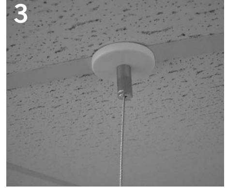
3 Secure non-feed canopy to 1/4-20 x 1 1/2" length stud (not provided) with threaded barrel.
