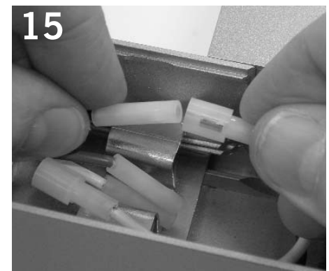
15 Connect like-colored electrical leads at power feed.
