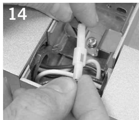
14 If applicable, connect like-colored electrical leads at joiner block at opposite end of luminaire body.
