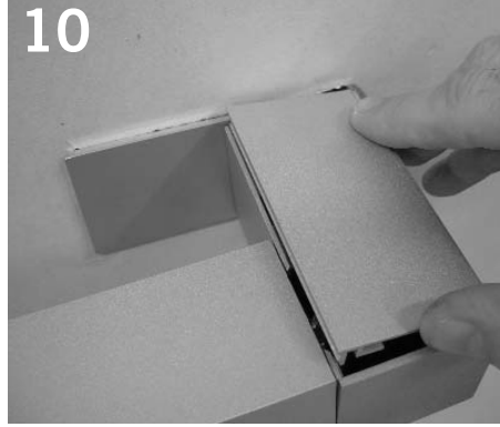
10 Snap end block covers into place. NOTE: Cover lip should face wall.
