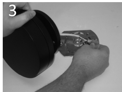
Make electrical connection while supporting fixture.
