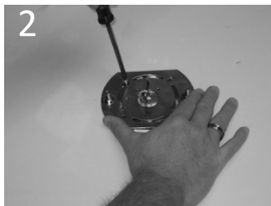
Run supply wires from wall through supplied mounting bracket and attach the mounting bracket to the octagonal J-box.
