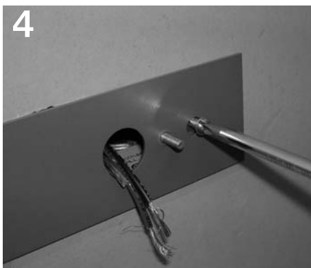
4 Anchor coverplate to j-box at one end and screw to wall at other end.
