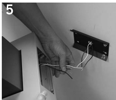
5 Make electrical connection.
