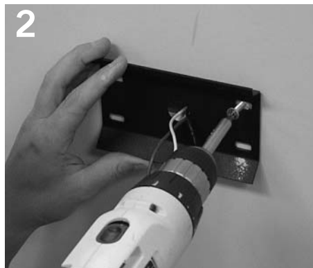
2 Attach mounting bracket to wall. NOTE: Fixture weighs approximately 15 lbs. Reinforce wall as required.
