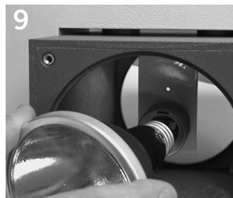
9 Install lamp per relamp label. Reinstall lamp coverplates.
