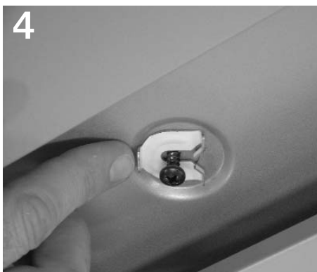
Raise fixture into place. Slide mounting clips over screws and tighten to secure fixture.
