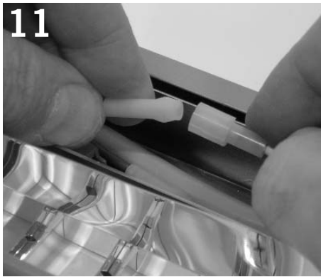
11 Connect node joiner cord to jumper wires inside splice compartment.
