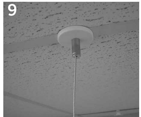
9 Secure non-feed canopy to 1/4-20 x 1 1/2" length stud (not provided) or caddy clip with threaded barrel.
