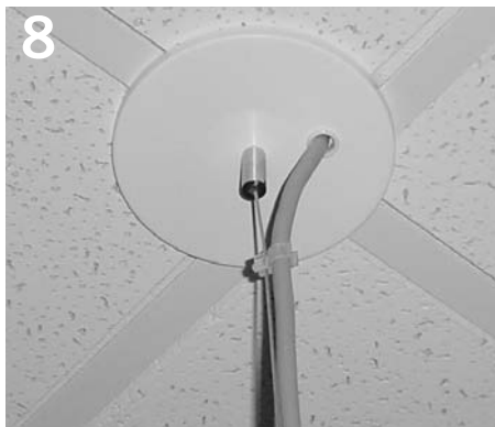
8 Secure feed canopy to 1/4-20 x 1 1/2" length stud with threaded barrel.
