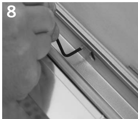
8 Level fixture by tightening allen screws.
