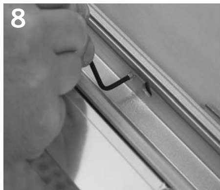
8 Level fixture by tightening allen screws.
