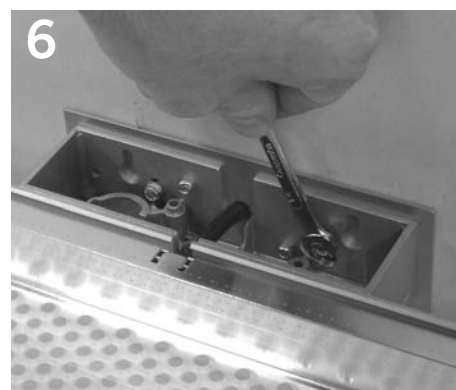
6 Tighten mounting screws to secure fixture to wall.
