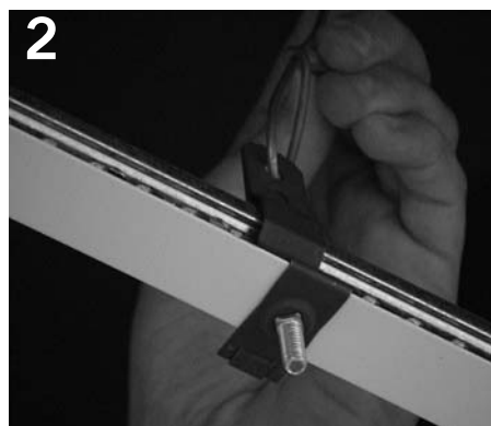
2 Wire fixture to deck above ceiling, according to local code.
