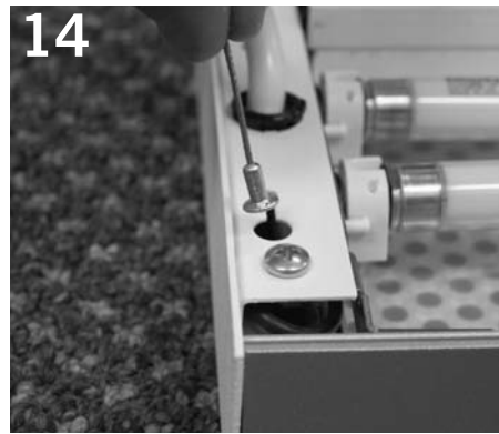
14 Slide hanging cables in eye-holes to hang fixture. Install lamp - 28 watt or 54 watt T5.
