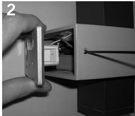
2 Loosen set screws and remove backplate from light.
