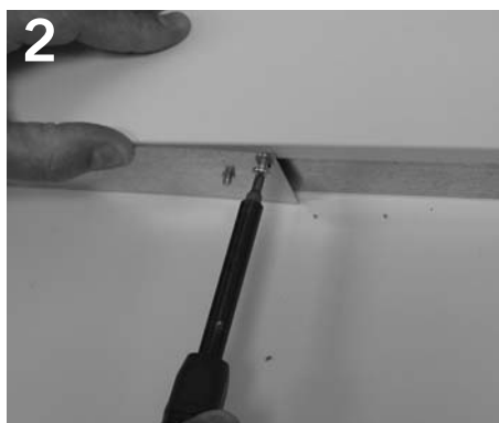
2 Unscrew panel on side of louver channel.
