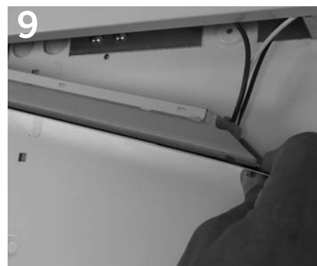
9 Remove panel to access ballast.
