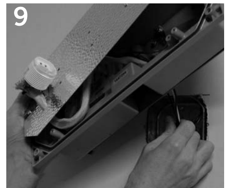
9 Make electrical connection and push wires back into junction box.
