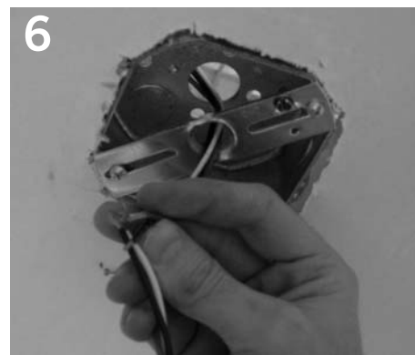
6 Complete electrical connection through center threaded hole in bracket bar.
