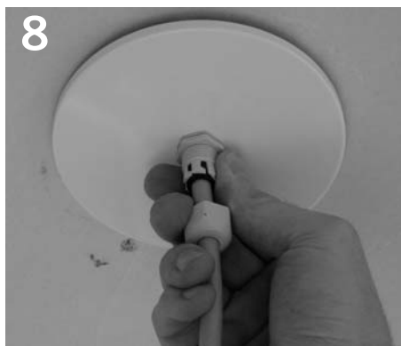
8 Thread compression fitting into center hole of bracket bar and tighten securely.
