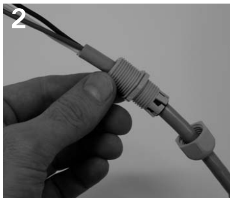
2 Slide compression fitting over power cord.
