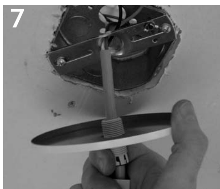
7 Push electrical connections into junction box through center threaded hole. Insert power cord into center hole.
