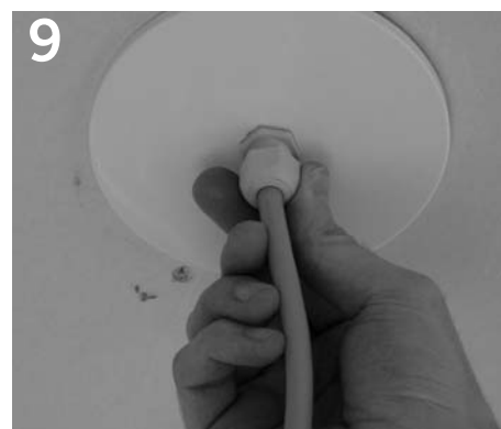
9 Tighten securing collar into compression fitting to secure fixture.
